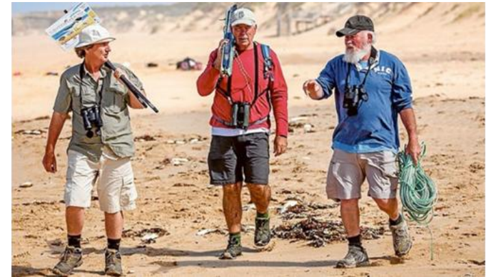
The effort to help hooded plovers breed successfully is well underway with Graeme Millar, Neil Shelley and Denis Goss constructing a protective barrier at Gunnamatta. Photo by Yanni
